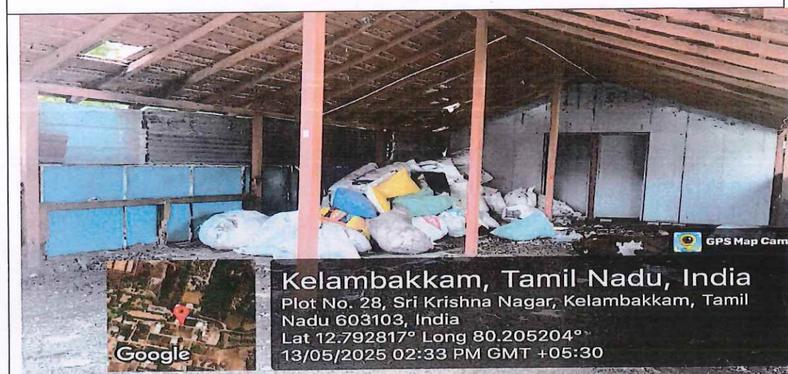
Shredded Plastic Waste Storage Shed
